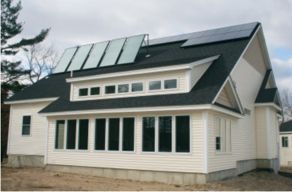
Left: Twenty-one photovoltaic panels on the south-facing roof generate about thirty kilowatt hours on a sunny day. The sun also heats fluid in five hydronic roof panels that deliver their heat to hot water storage tanks in the partial basement.
